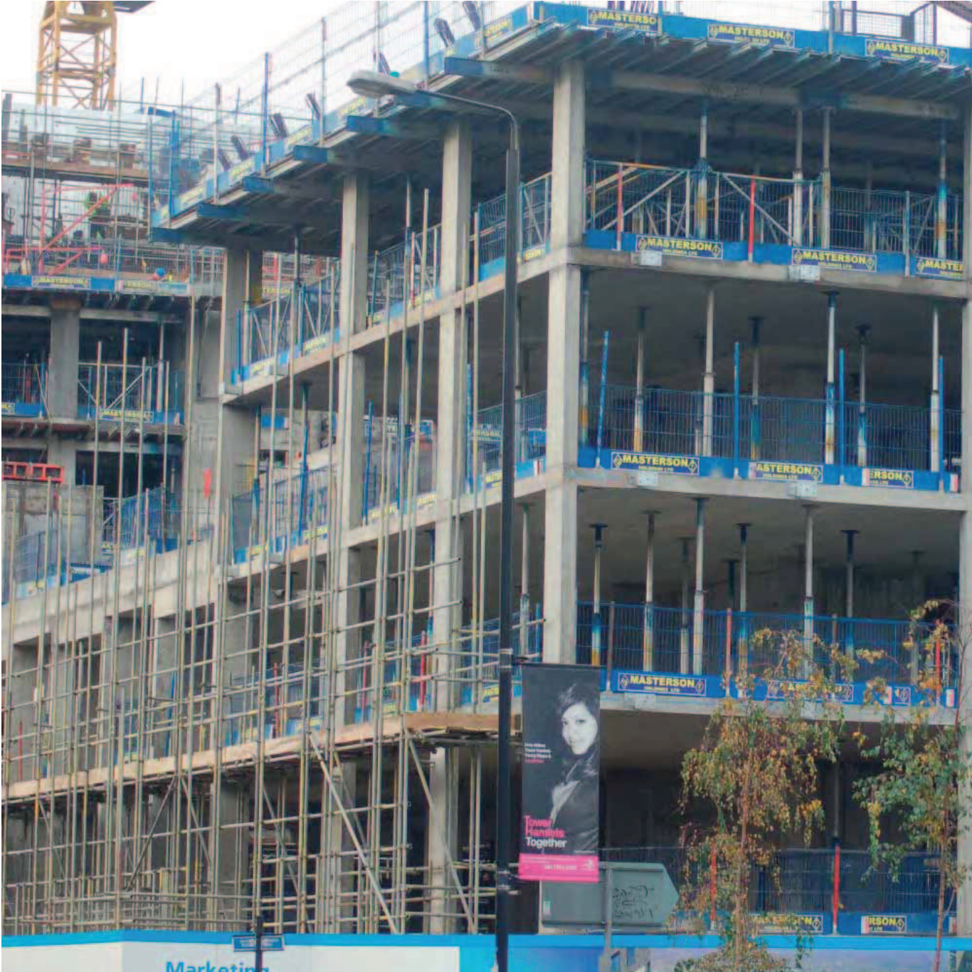
St Andrews under construction
