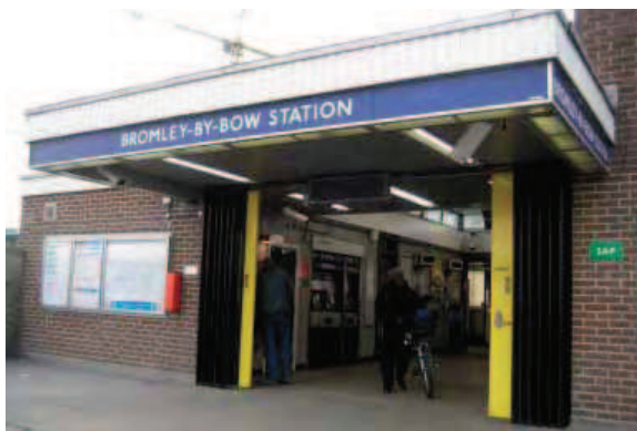
Significant opportunities exist to improve the experience of arrival at Bromley-by-Bow Station
